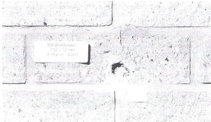
Figure 4 - Damage to concrete brick caused by .308 Winchester
